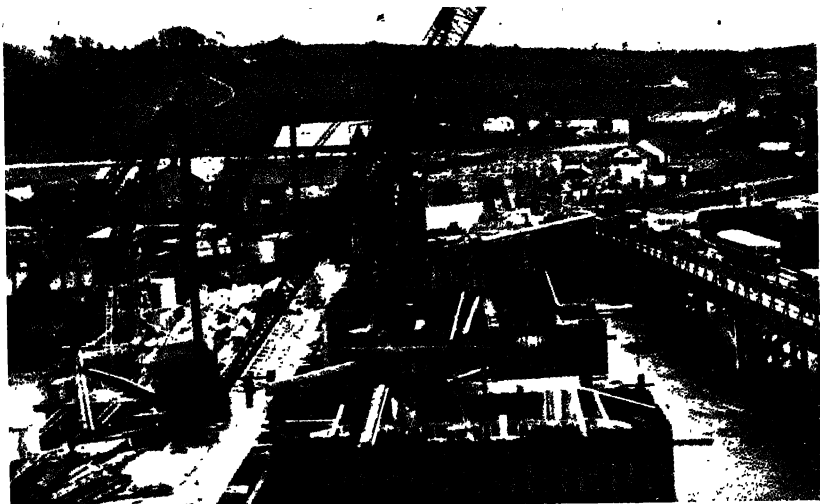
Fig. 274.—Bridge Construction from a Working Stage.
